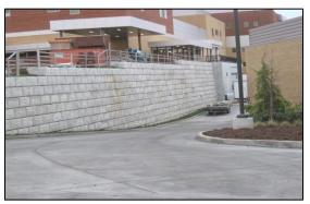
The project presented some challenges related to wall engineering. Wall heights of approximately 28 feet tall, seismic considerations, as well as significant loading from the actual hospital structure all needed to be well thought out. Time was critical and the start of building construction was dependent on the StoneTerra wall installation.
